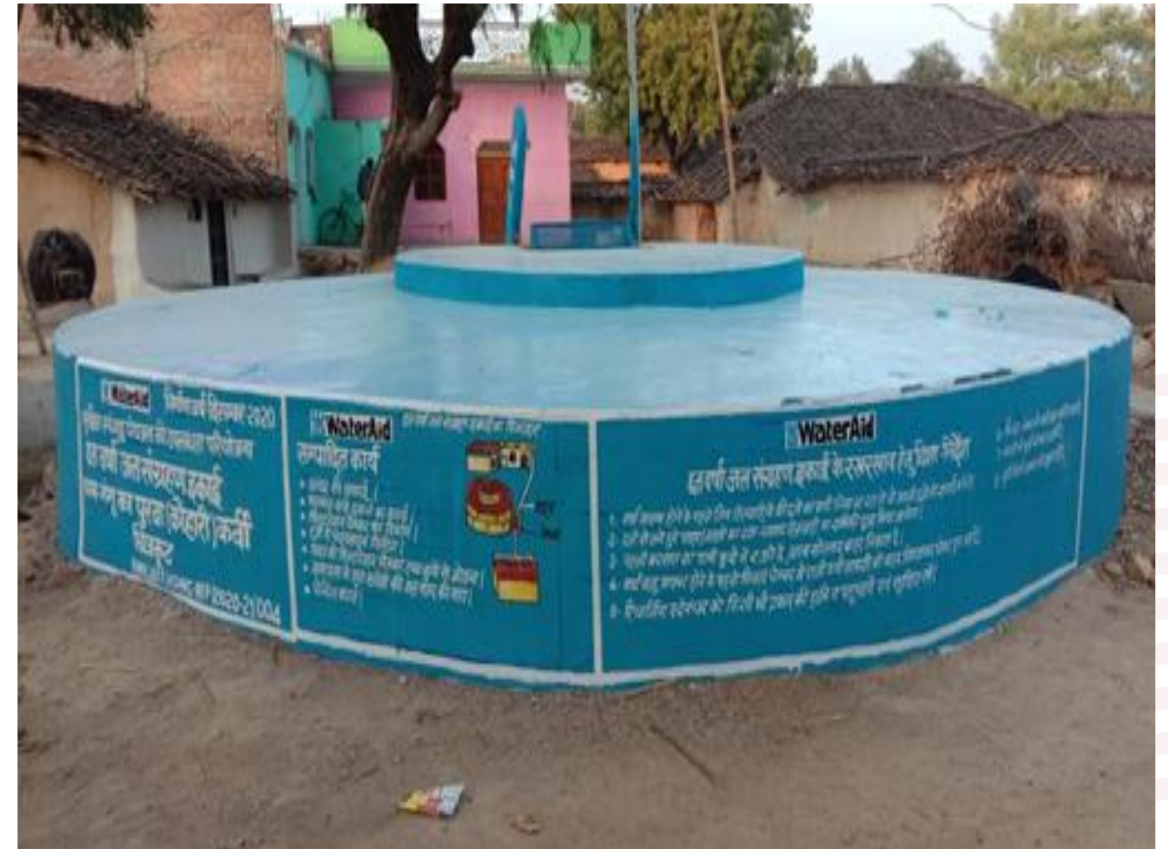
Rainwater Harvesting Structure
